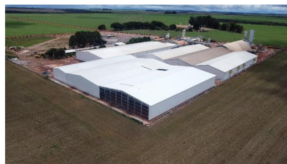
Construction in Progress / In Conclusion
