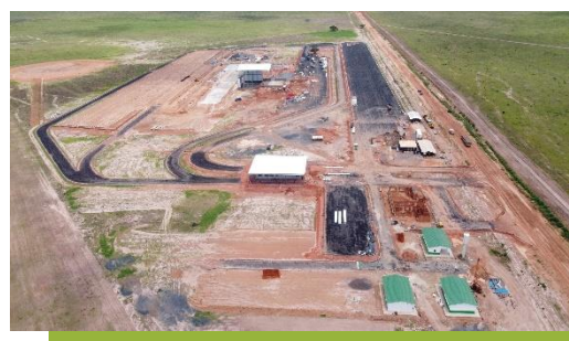
Constructions in Progress
